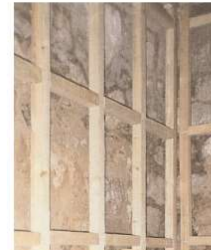
Fig71: Stone Wall with Timber Studding (BRE, 1999)
