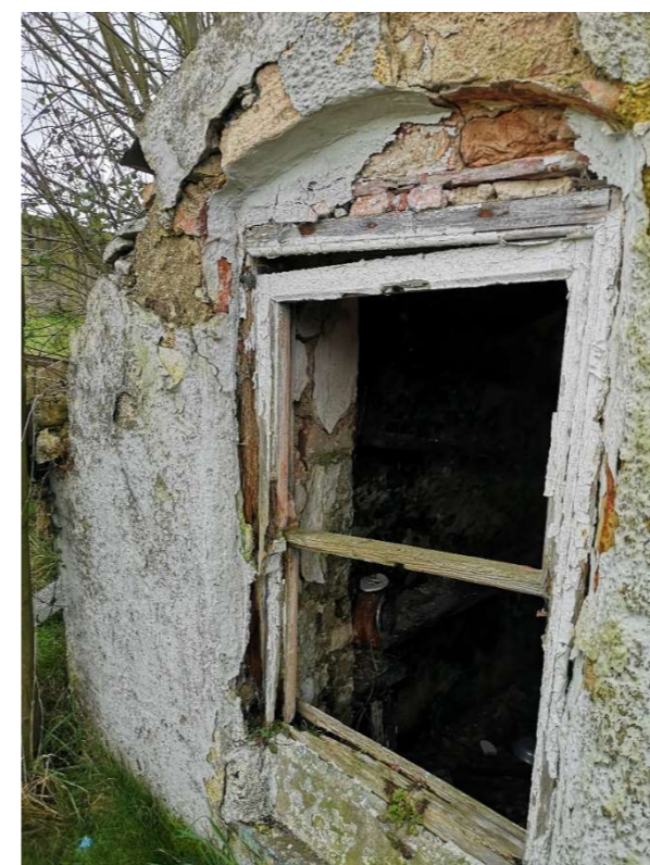
Fig53: Window Condition 2 (Author, 2021)
