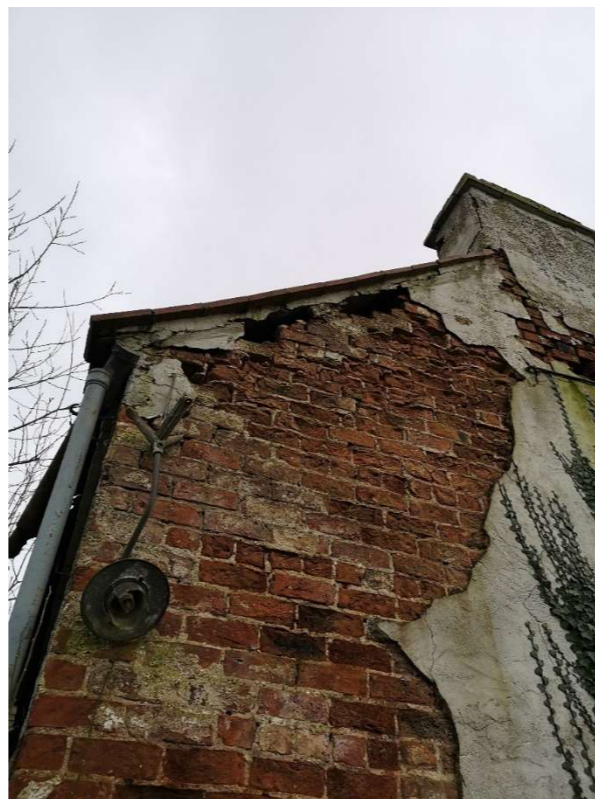
Fig56: Wall Condition 1 (Author, 2021)
