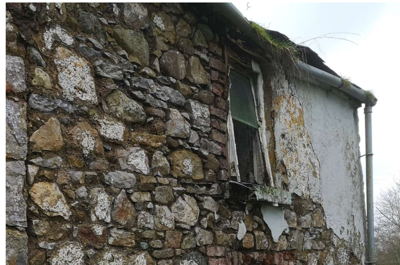
Fig52: Window Condition 1 (Author, 2021)
