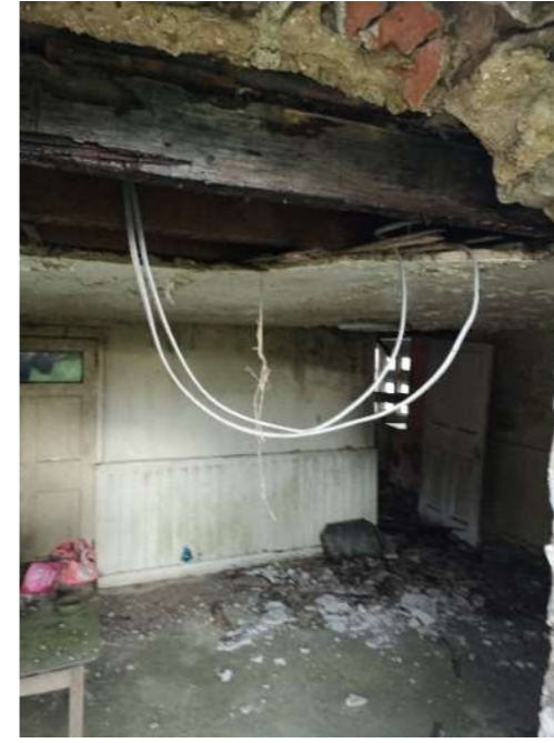
Fig18: Floor Joists (Author, 2021)
