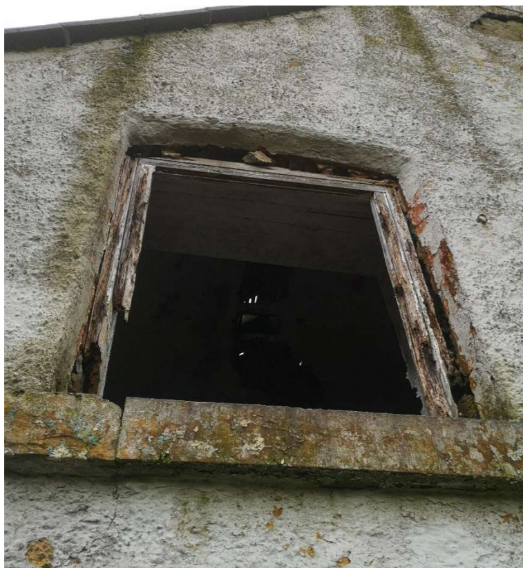
Fig67: Window Condition (Author, 2021)
