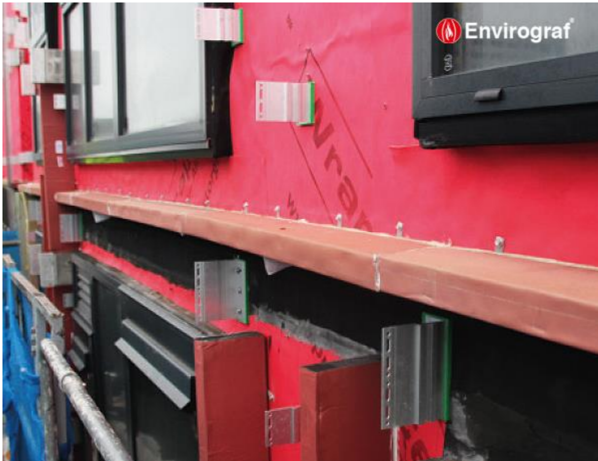
Fig12 – Cavity Barrier (Envirograf, 2021)
