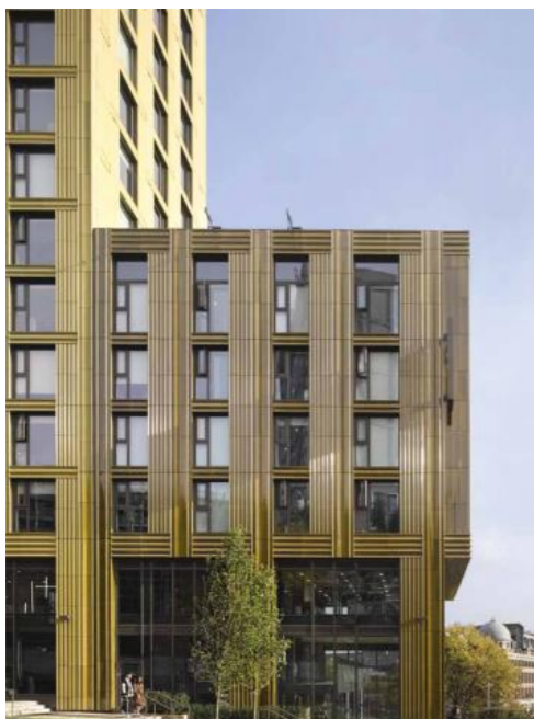
Fig39 - NBK Façade Building (NBK, 2021)
