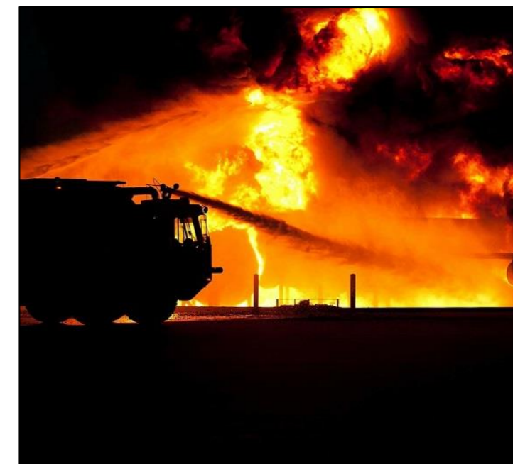
Fig98 - Building Fire (Designing Buildings Wiki, 2021)
